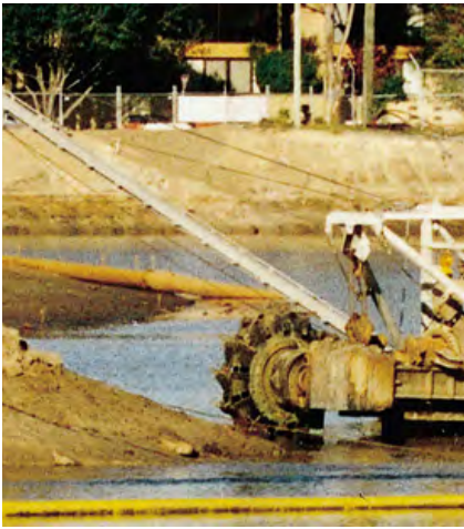
Figure 126.1 Dredge in new Gold Coast canal estate Bob Moffatt
