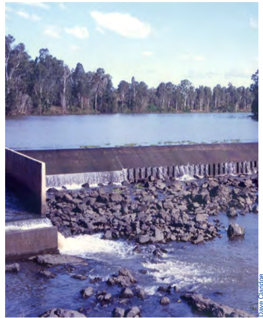
Figure 115.1 Barrage - a river impoundment
