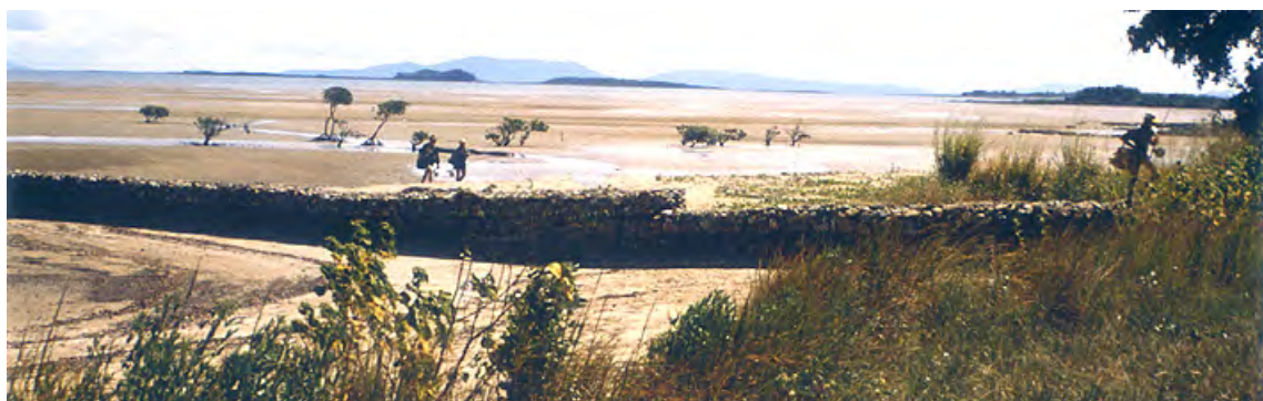
Figure 113.1 Bund walls such as this close off areas of coastal wetlands, causing major changes in the ecology of the area and long term changes to fish stocks.
